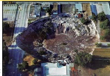
Giant sinkhole in Winter Park, Florida.
