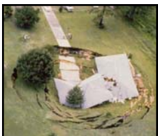
House collapses into sinkhole.
