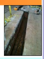
While the floor was opened up, we ran two water feeds from the main tunnel to the vacuum area
