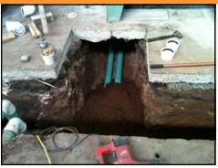
A trench was dug to install better drain lines from the vacuum area and 389-399 tanks to the tower and waste water pits and also to install cooling lines from 952 chiller to 389-399 tanks.
